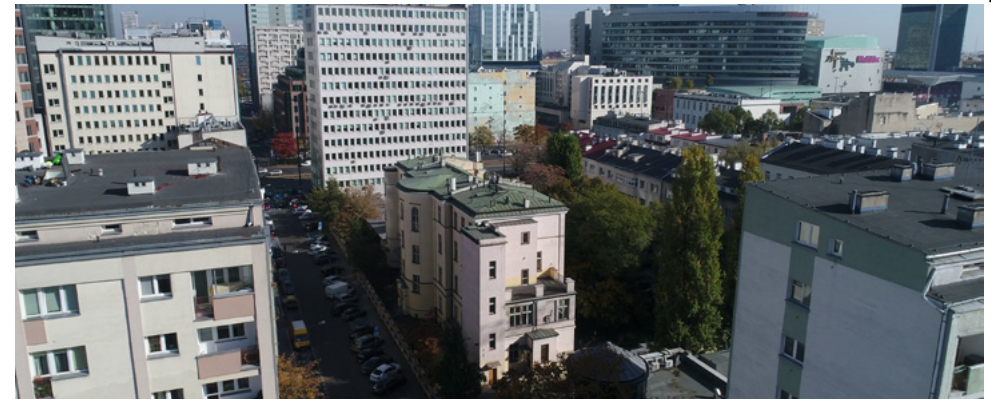
Bersohn and Bauman Children's Hospital. Photo WGM
